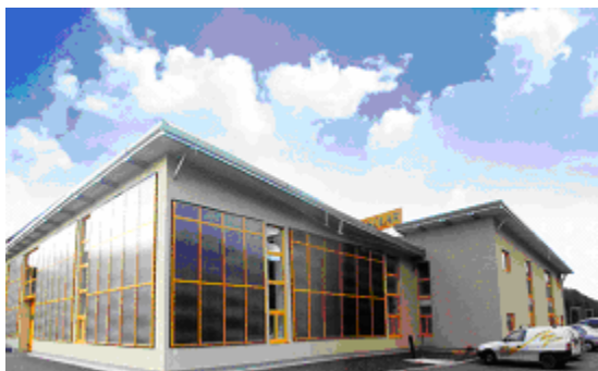
Solar-heated factory building of the collector manufacturer SIKO in Austria
