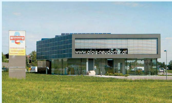
This warehouse with an integrated office building is an HVAC installation firm in Austria. It has solar thermal collectors installed on the roof for space heating the warehouse and offices and façade-integrated photovoltaic panels for electricity. The section of the building containing the offices is built according to the 'Passivhaus' standard with an annual space heating consumption of 18 kWh/(m<sup>2</sup> a). The warehouse is equipped with an underfloor heating system.
